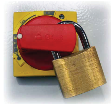
Fig. 44 Securing the main switch
